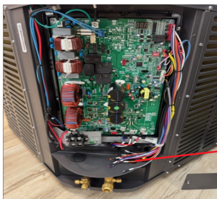
Figure 11.4B- 24V Control Terminal Connections
