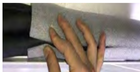
Figure 7.8A - Insulation and Deadening Pad Applied to Indoor EZ-Fast CONNECT™ Joint
